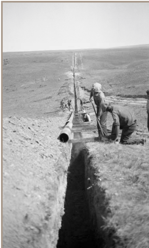
Digging Pipeline, Turner Valley, Alberta, 1929
