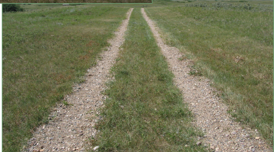
Reclaim and Reduce Disturbance During Operations: Two Strip Graveled Surface Minimizes Soil Disturbance and Provides Year Round Access
