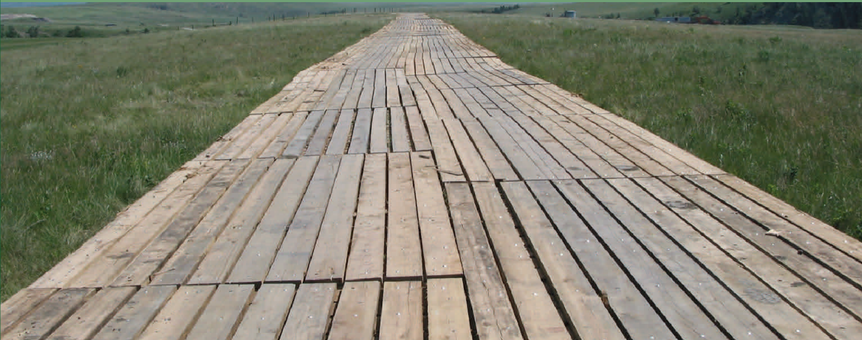
Temporary Access Using Interlocking Matting
