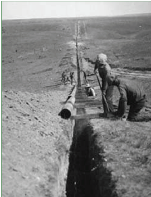
Early Pipeline Construction
