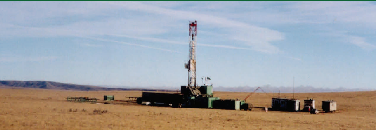
Reduced Disturbance Wellsite Construction, Cypress Hills
