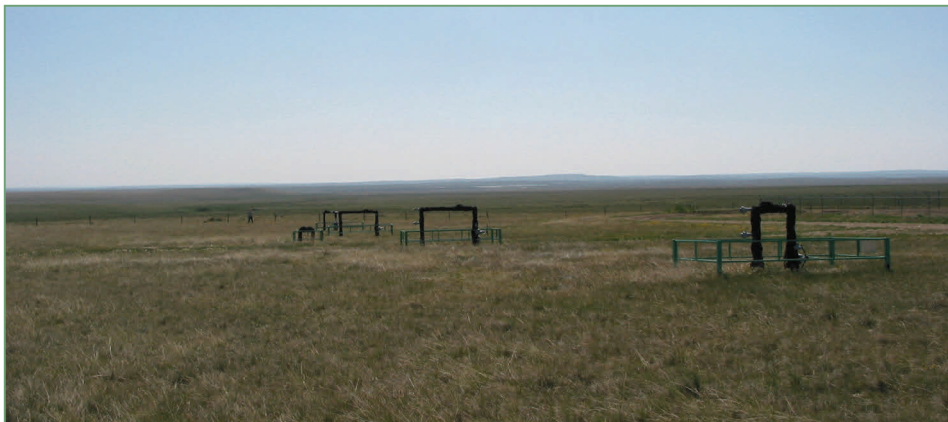
Cluster Development: Multiple Flow Lines in a Common Corridor, Multiple Well Bores from a Single Well Pad, Cypress Hills
