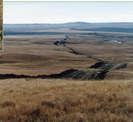
Cypress Upland Ecodistrict Pipeline Construction
