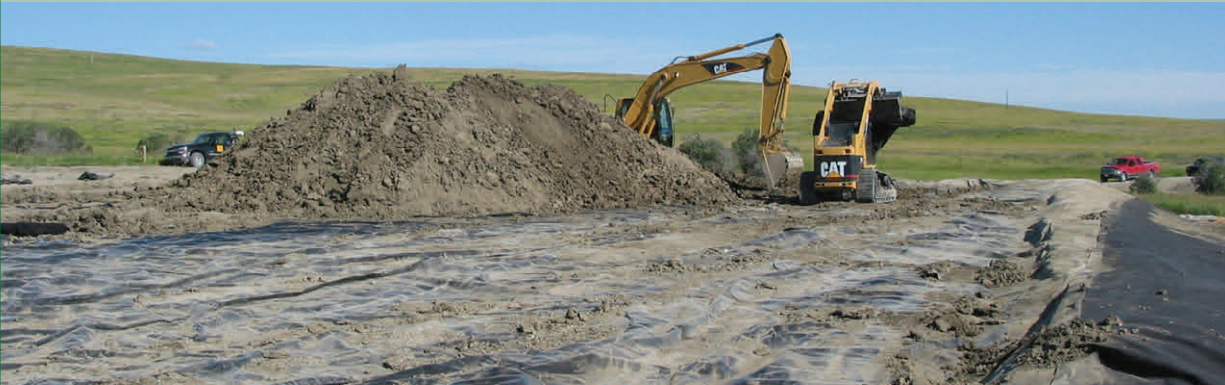
Use of Barrier Fabric to Conserve Surface Vegetation, Trained Operators with Experience are Key to Success
