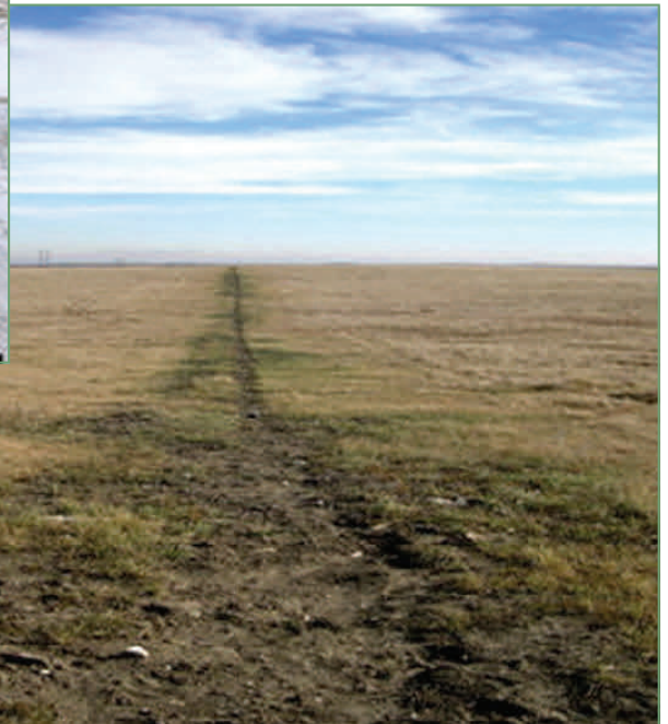
Minimal Disturbance – No Strip Pipeline Construction Operates on Frozen Ground Conditions, Majorville
