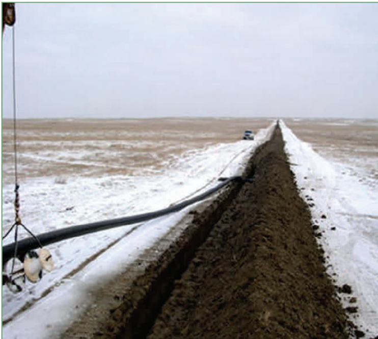
Minimal Disturbance – No Strip Pipeline Construction Operates on Frozen Ground Conditions, Majorville
