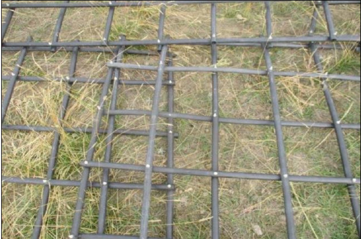
Figure 9. Livestock deterrent panels used to protect a reclaimed wellbore. Photo courtesy of Joel Conrad, Salix Resource Management Ltd.
