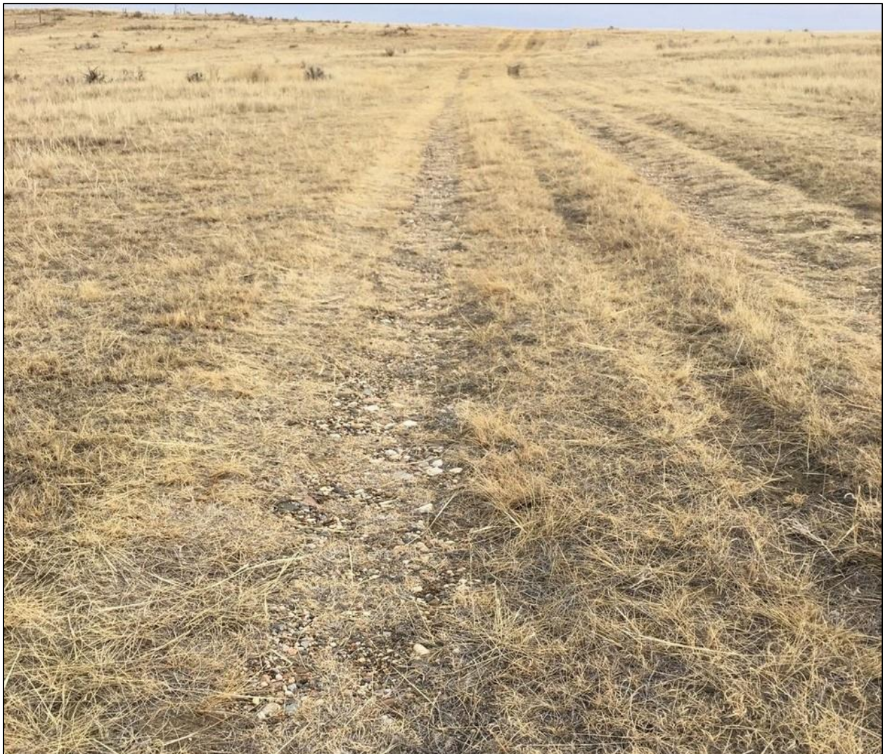
Figure 2. Soil compaction, rutting and trail braiding on a two track gravel access trail in DMG. Photo courtesy of Nolan Ball.
