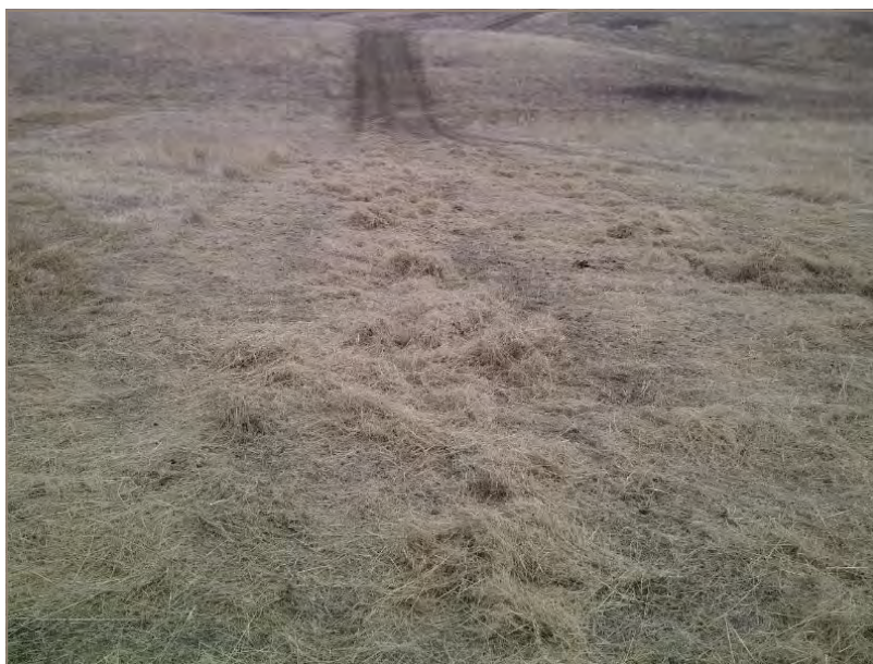
Wild Harvested Hay Spread on Exposed Topsoil on a Narrow Linear Disturbance
