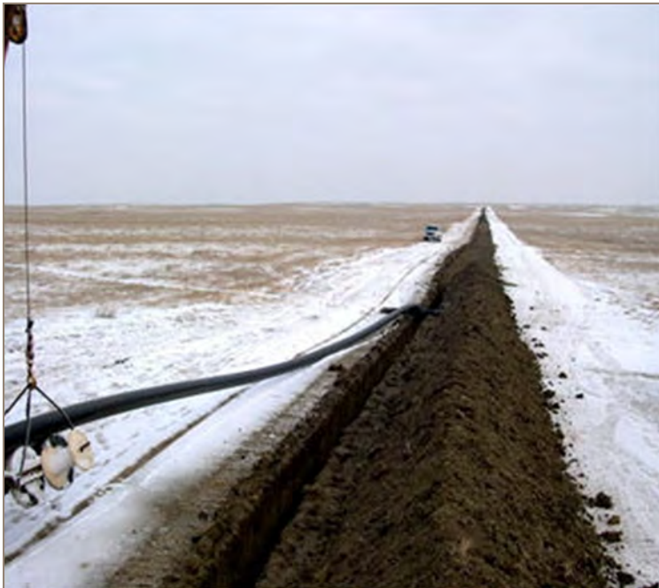
Minimal Disturbance Pipeline Constructed During Frozen Ground Conditions With No Soil Stripping
