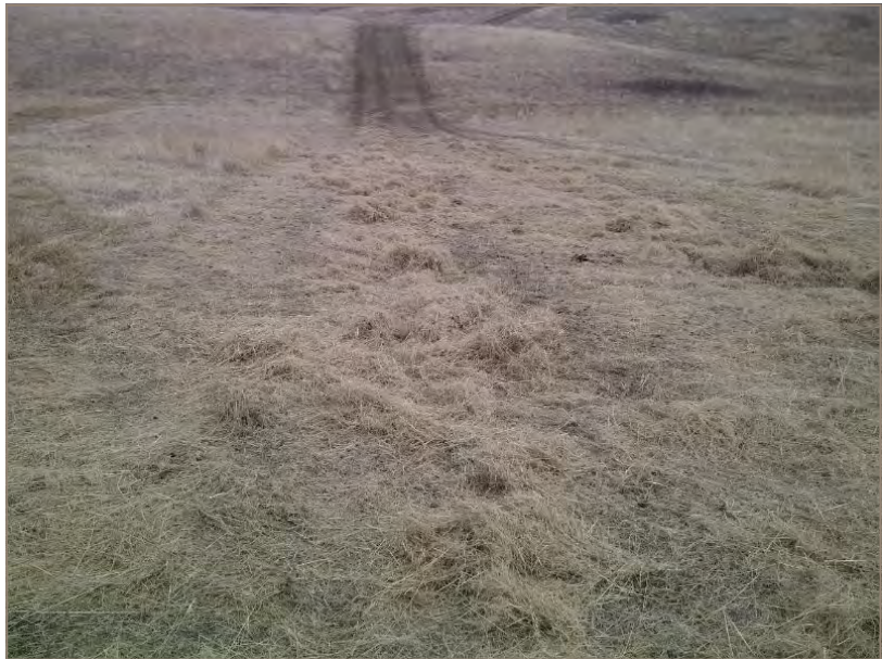
Wild Harvested Hay Spread on Exposed Topsoil on a Narrow Linear Disturbance
