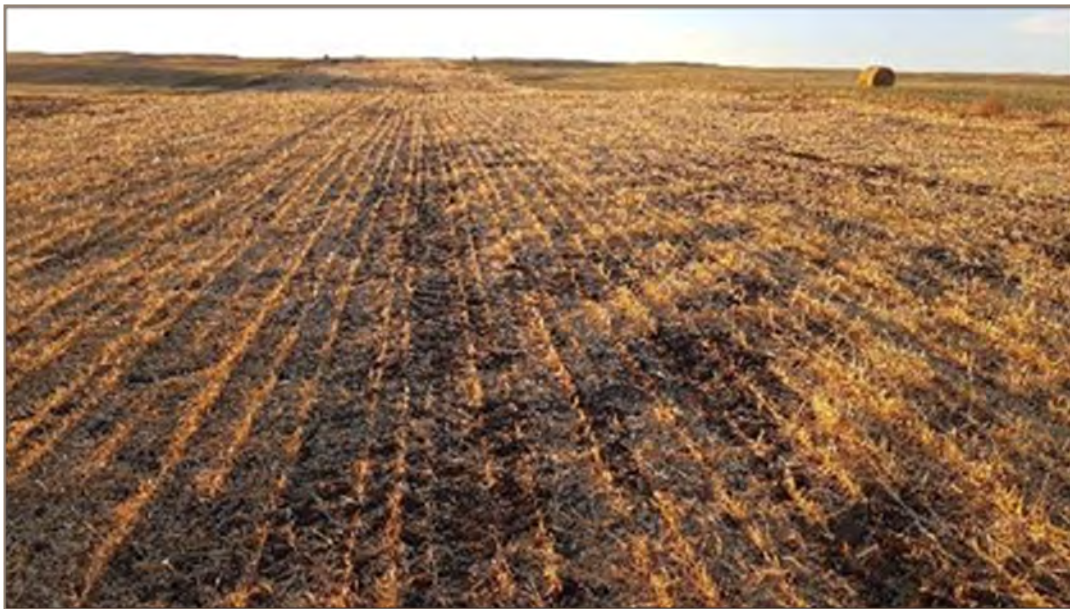
Straw Crimping to Mitigate Erosion Potential and Shelter Seedlings on a Large Surface Disturbance
