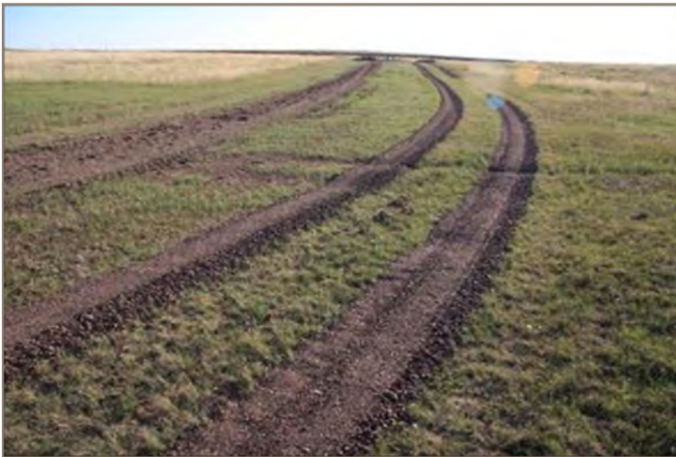
Newly Constructed Flow Line and Adjacent Two-track Gravel Access Trail
