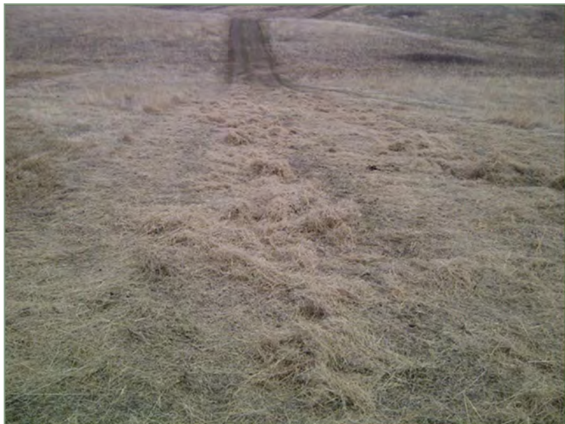
Wild Harvested Hay Spread on Replaced Topsoil - Pipeline RoW
