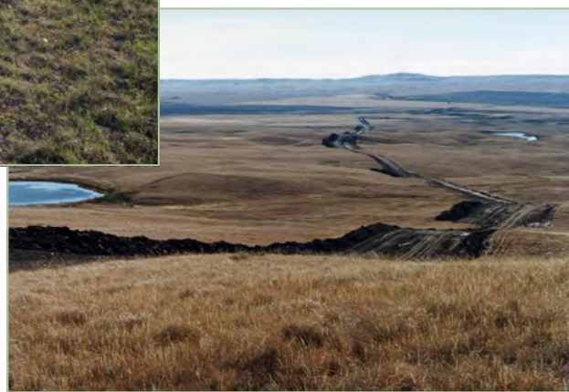
Cypress Upland Ecodistrict Pipeline Construction
